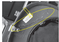
FIG. 10 Major Structural Crack
